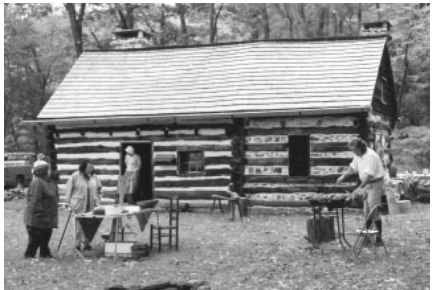
Lower Swedish Cabin, Creek Road, Drexel Hill, PA
