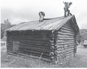
Dismantling the threshing barn, June 2017. (Photo by Joseph Mathews)
